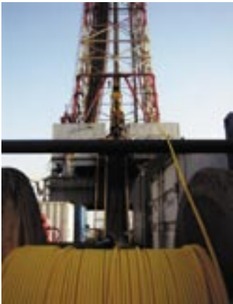
Installation of encapsulated tubewire.
